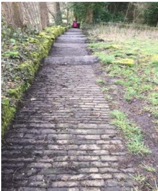
In Sowerby this fine setted path at the back of Ryburn Valley High School was covered in mulch with encroaching brambles
