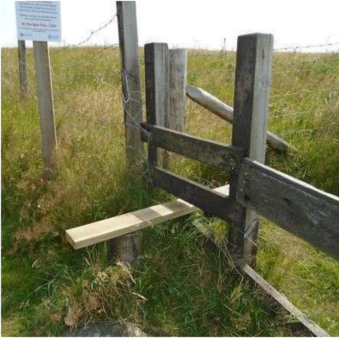
An example of the many stile repairs we have done this year. This is one just needing a new tread-board was at Keb Hill was funded by Todmorden Town Council.
