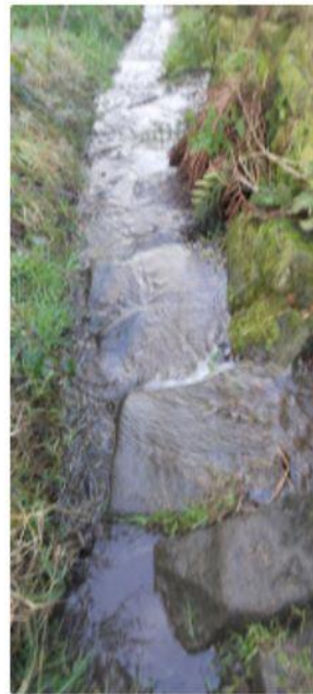
A lovely causey path near Wood Top, Cragg Vale . The water was taken off the path by digging out the channel. Work funded by Hebden Royd Town Council Mayor's fund.
