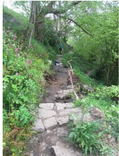
A landslide on the path to Hebble Hole made the path unstable. We widened the path and put in hazard tape. Work funded by Calderdale Highways (who have now installed a boardwalk)
