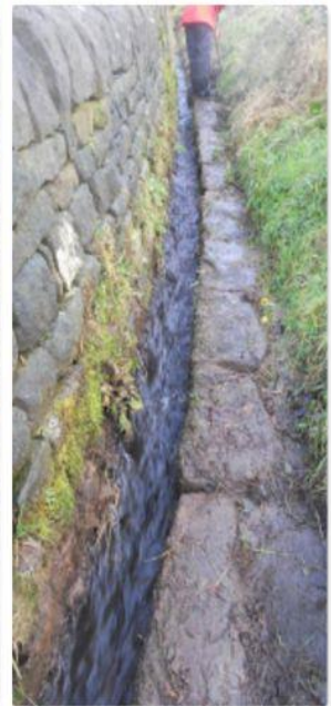
A lovely causey path near Wood Top, Cragg Vale . The water was taken off the path by digging out the channel. Work funded by Hebden Royd Town Council Mayor's fund.
