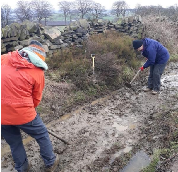
Scraping a path at Krumlin
