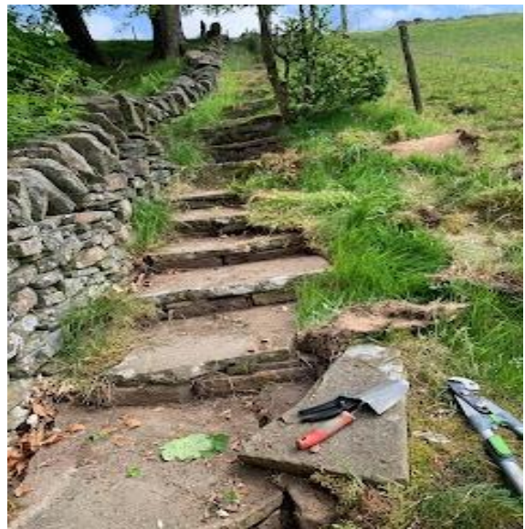
Widening steps at Mill Bank.
