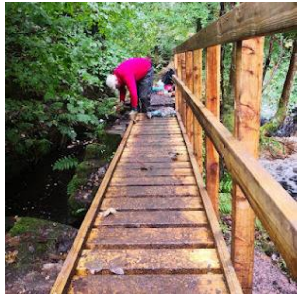
Bridge replacement in Cragg Vale.
