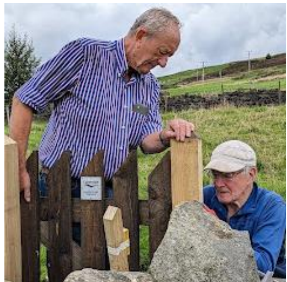
Fitting a gate at Old Town.
