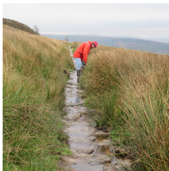
Drainage work on a causey path at Whirlaw.
