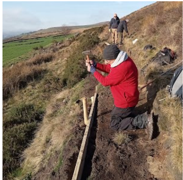
Securing a path edge at Midgley.
