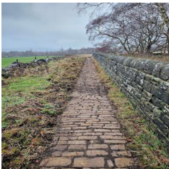
Path clearance at Longley Lane, Ryburn.
