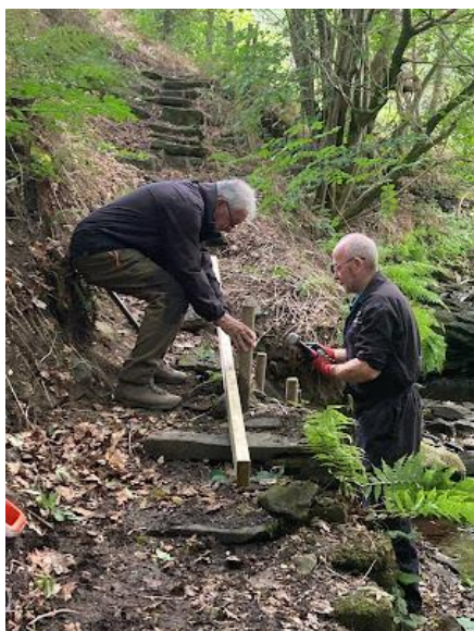
Revetment in Luddenden.
