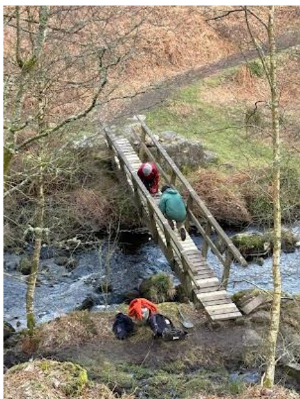
Bridge repair at Blake Dean.
